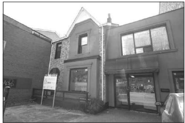
Below: 1894 Yonge Street, squished between more modern buildings, all destined for redevelopment.
